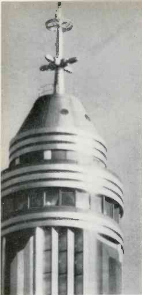
WNBT - W2XWG ANTENNAS. Lower turnstile elements simultaneously transmit television pictures and FM broadcasting without mutual interference
